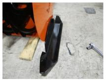
4) Securely fasten the Skid-Skis to the Snow Blower collector housing using the hardware provided. Insert the fasteners such that the flat head of the carriage bolt is inside the collector housing and the washer and nut are on the outside of the collector.
